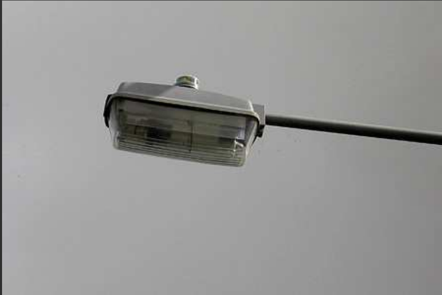
Old style, very prevalent, exposed luminaire, blinds onlooker, causes light pollution, wastes energy
